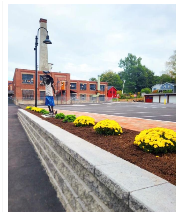
Municipal Parking Lot Improvements
