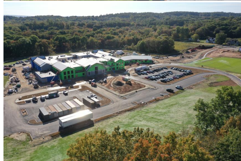
Top: Construction of the New Norton School Bottom: Construction of the new Barnum School Source: Cheshire BoE
