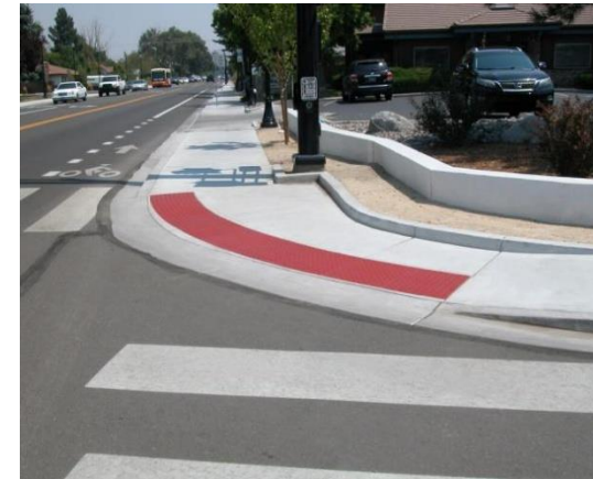
Above: Accessible Sidewalk Ramp
